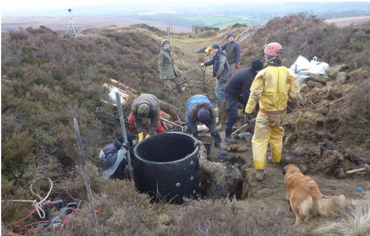
Installing the pipe into the new shaft entrance dropping into the adit.
