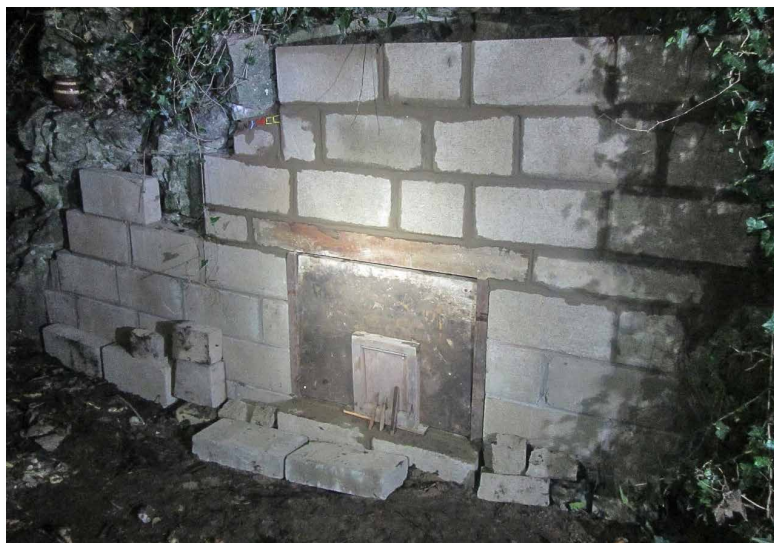
The one-way door installed into Manor Vale East Cave to allow the badger to leave without re-entering the cave.
